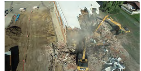
Clafin Excavating taking down the historic structure.
